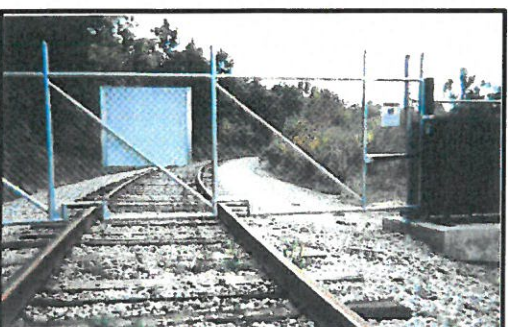
Custom Curb Notch
